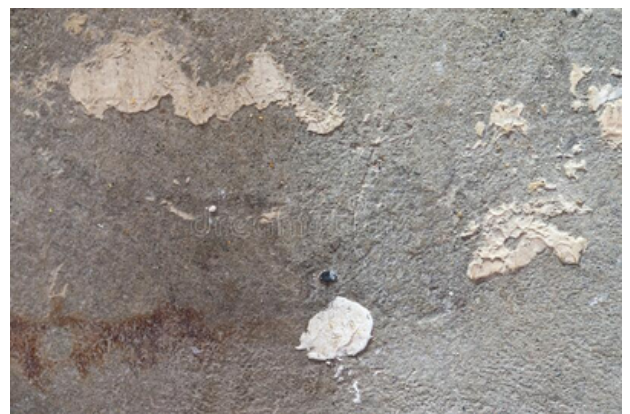
Adhesive contamination of concrete sub-floors
